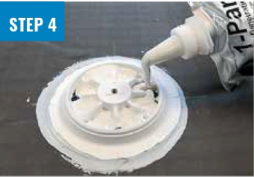
FILL WITH CHEMLINK 1-PART & PLACE CAP
